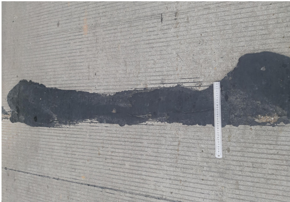
Tambalan Kecil ( Patching Small )
