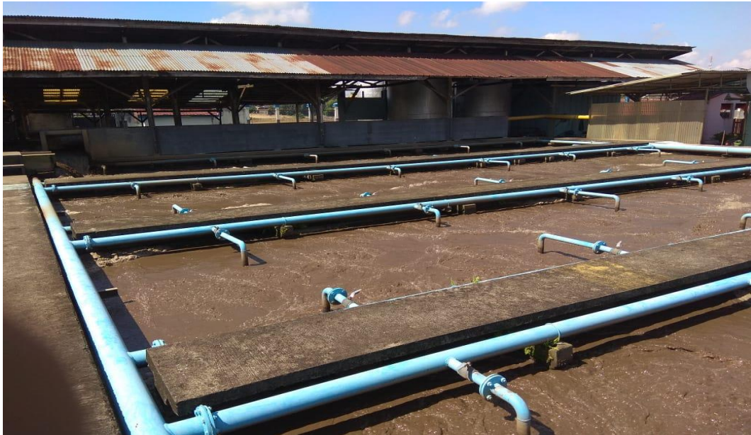
Gambar 4.10 Bak Pengolahan Completely Mixed Activated Sludge (Aerasi) (Dokumentasi Lapangan,2021)
