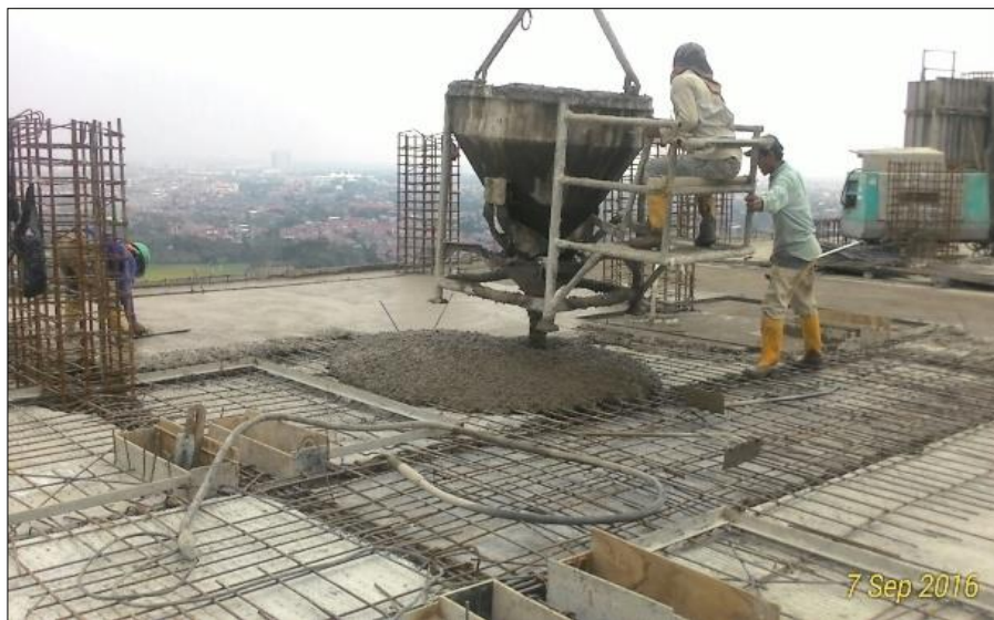
Gambar 2. 6. Pengecoran Cast In Place Sumber : SIBIMA Konstruksi (2019)
