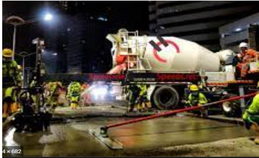
Gambar 2.13 Pengecoran Speedcrete Holcim
