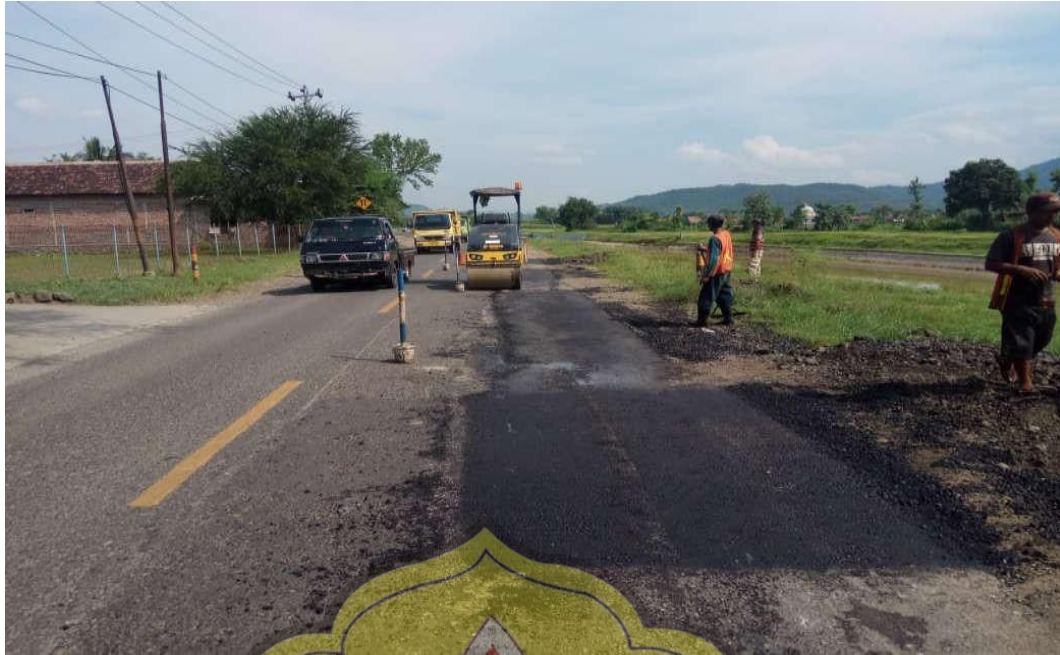
Gambar 2.17 Tambalan ( Patching end Utiliti Cut Patching )
