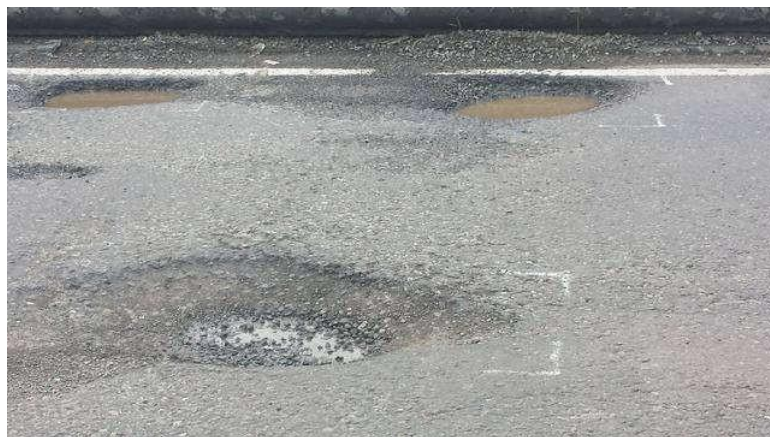
Gambar 2.18 Lubang ( Pathole )
