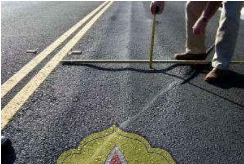
Gambar 2.20 Alur ( Rutting )
