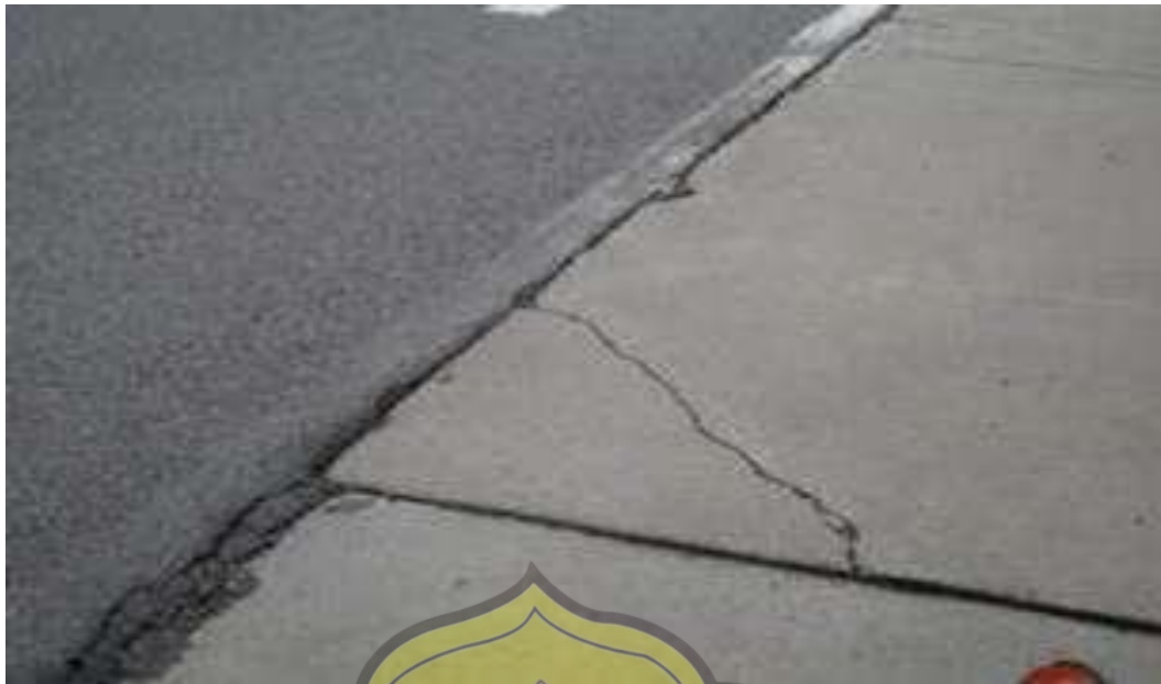
Gambar 2.14 Retak Sambung ( Joint Reflec Cracking )
