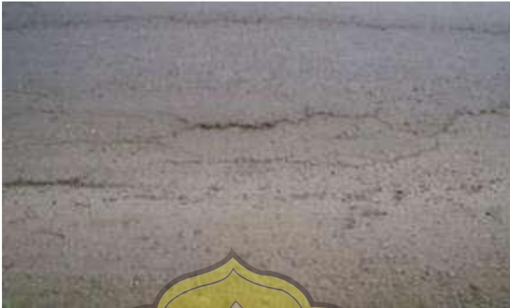
Gambar 2.8 Cekungan ( Bumb and Sags )
