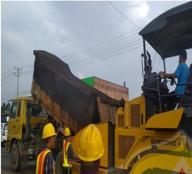
Gambar 1. Loading aspal panas *aspalt finisher*
