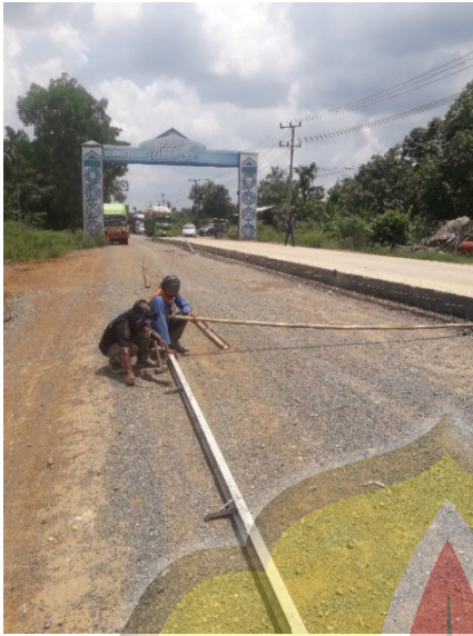
Pemasangan Mall Bekisting Lean Concrete (LC)
