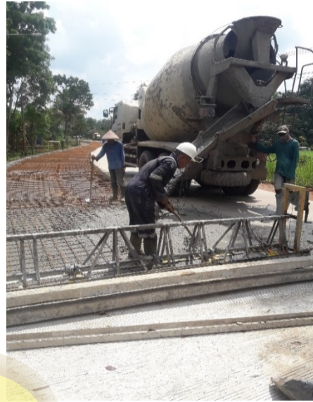
Proses Penghamparan Beton Ready Mix
