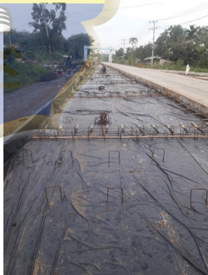
Pemasangan Plastik diatas Beton Lean Concrete (LC)
