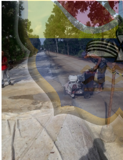
Proses cutting jalan rigid
