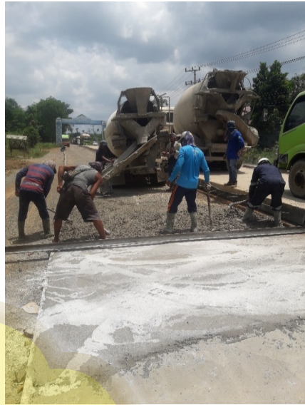
Proses Penghamparan Beton Lean Concrete (LC)
