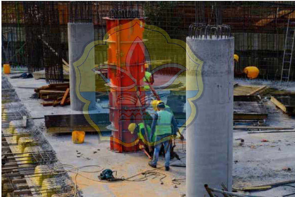
Gambar 2. 3 Bekisting Fiberglass
