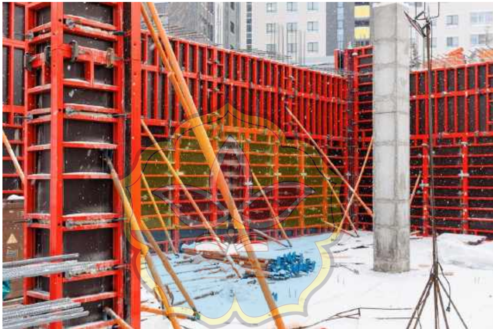
Gambar 2. 2 Bekisting Semi Sistem
