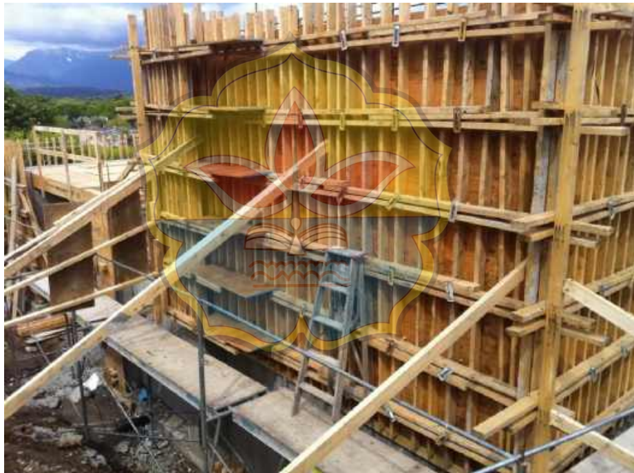
Gambar 2. 1 Bekisting Konvensional
