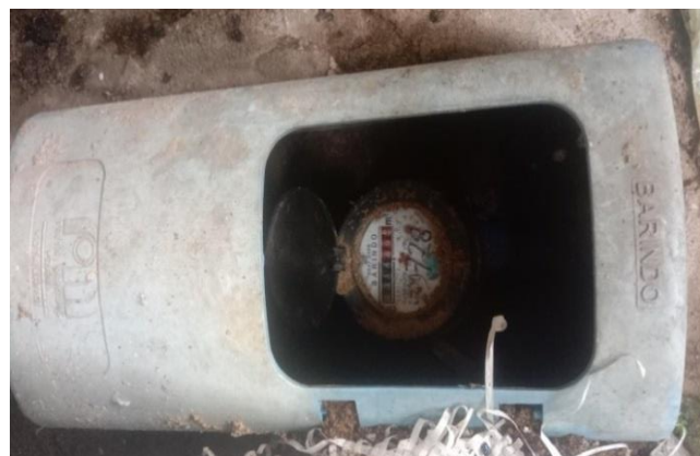
Gambar 4.1 Meteran Air PDAM
